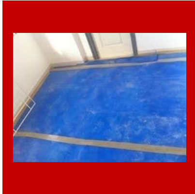
Tile Protection Sheet
