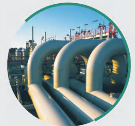
■ West- east gas pipeline
