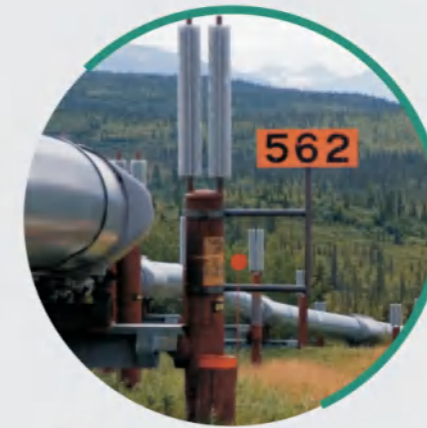
■ Pipeline for NICO
