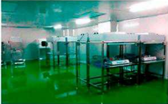
Meiri purification and fitting workbench (in CHN ENERGY STK# 001289)
