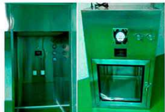
Meiri Purification Negative pressure weighing chamber and Laminar pass box (in Taitai Pharmaceutical STK#600380)
