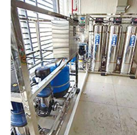
Yunnan Airport Large Water Purification Project
