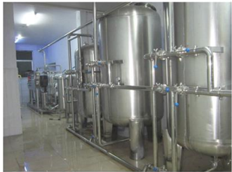
6T/H Double-stage RO equipment (high configuration)
