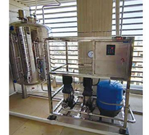
Frequency conversion constant voltage system in a community in Dongguan
