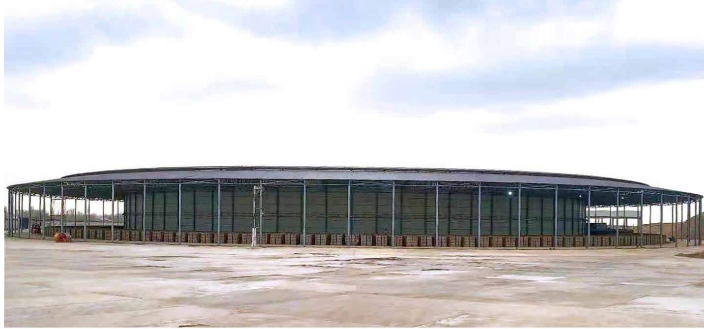
Project: Uzbekistan Rotary Kiln Location: Tashkent Kiln Section: 12.98m Kiln Capacity: 800,000 bricks /day Materials: mountain earth, coal gangue
