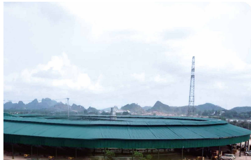
Project: Huang Gui Brick Factory Location: Huang Gui, Vietnam Kiln Section: 11.8m Kiln Capacity: 400,000-500,000 bricks /day Materials: shale, river sludge, construction
