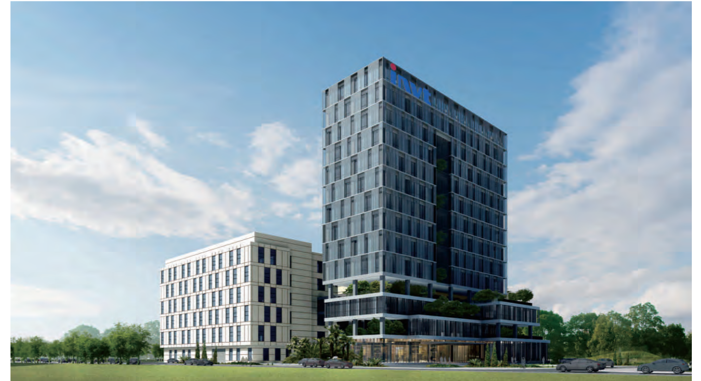
Shenzhen Industrial park
