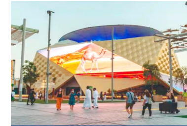
Outdoor Curtain Wall
