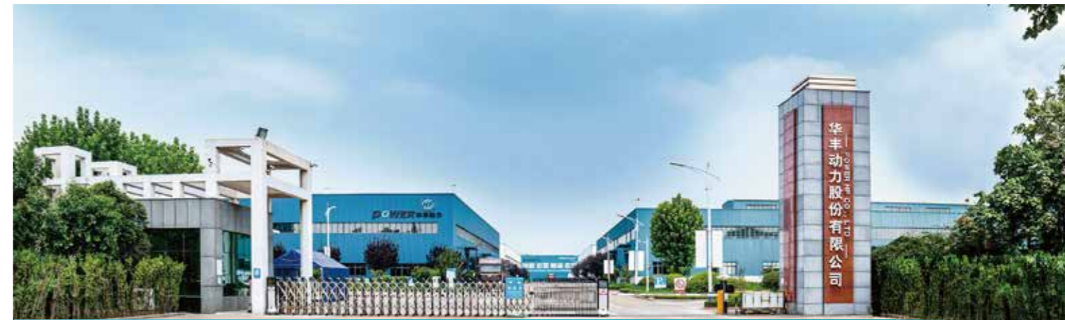
GENERATOR SET PLANT
