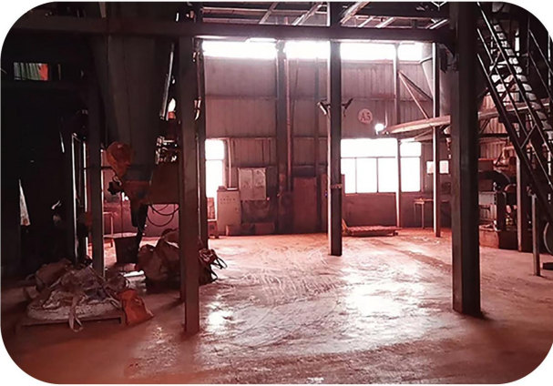
生产车间 Iron oxide red production workshop
