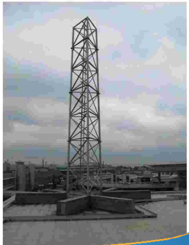
ROOF TYPE RADIO TOWER ISTANBUL AIR-PORT / TURKEY
