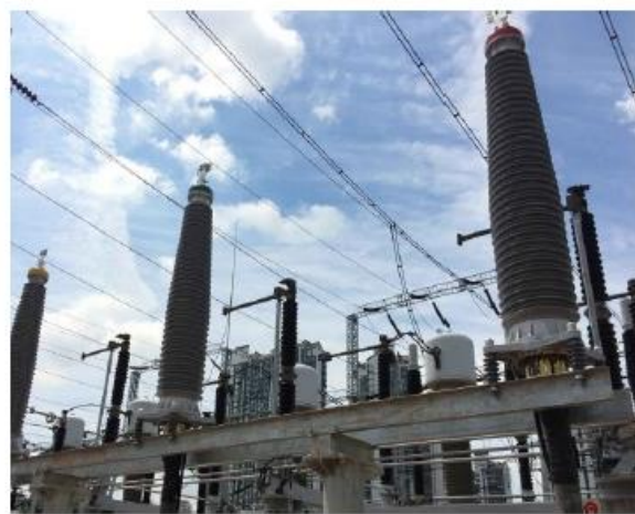
Zhuhai 220kV Fengji Line power transfer project
