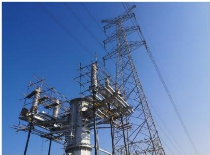
Quanzhou Fuxia DK170-880 220kV Luo Xin One And Two Road Project
