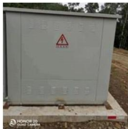
Anhui Suzhou 48.3MW Xiangshan Wind Farm Project
