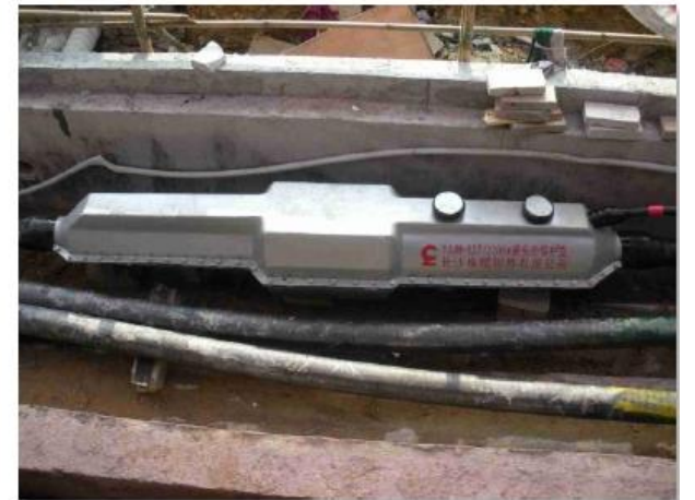
Guangzhou Wu-Guang Railway 220kV cable project
