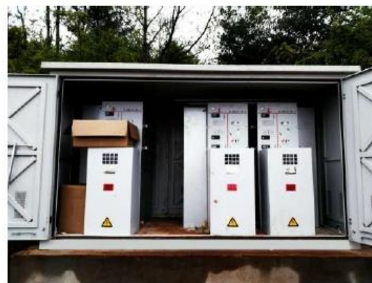
Yunnan International Dajipo (Phase III) 144MW wind power plant project
