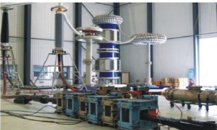
230kV cable and accessories test circuit
