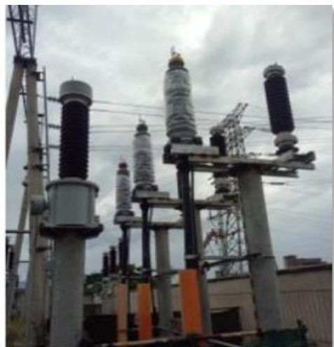
Chihu - Shilong 110kV cable project
