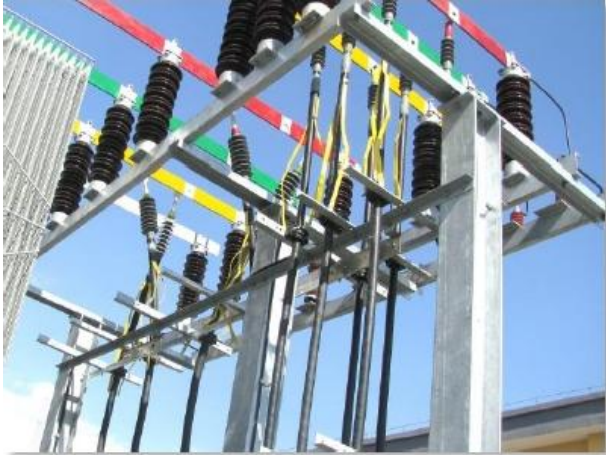
Harbin passenger special Changchun West Station cable project
