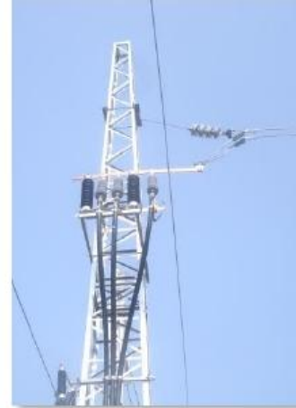
Beijing-Kowloon Railway Electrification transformation project
