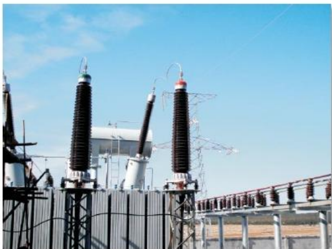
Liaoning Fuxin wind power 220kV cable project
