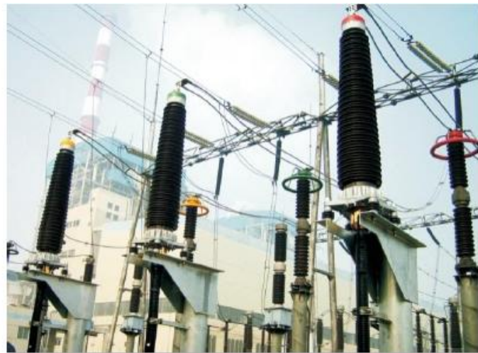
220kV cable project Huarun Thermal Power Plant in Nanjing, Jiangsu Province
