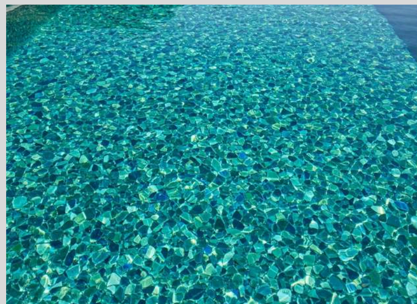
Swimming Pool Tiling
