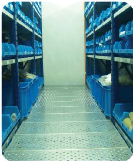
Steel Plank Flooring
