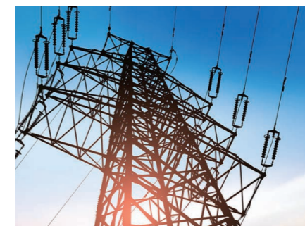
应急电力系统/Emergency Power System
