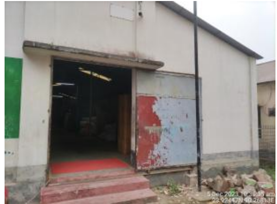
Shed-3 Raw material and Cutting section.jpg
